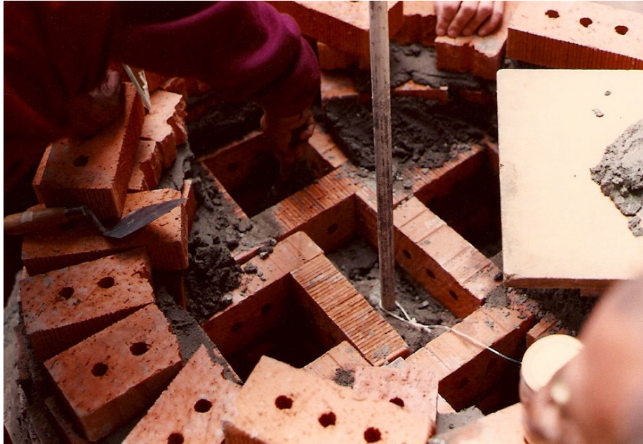
Figure 12: Finishing The Relic Chambers
